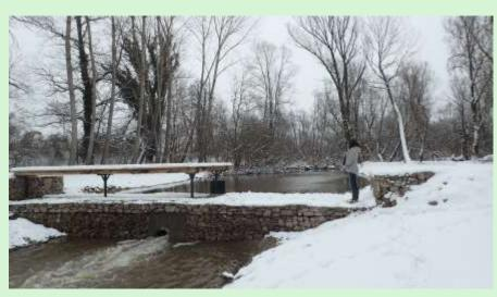
fill up the oxbow. Close to the bottomewier a fishpath has been constructed to help the migration of certain fish species. To prevent the erosion the core of the artefact was built by concrete, but it was covered by stone to fit into natural environment.
